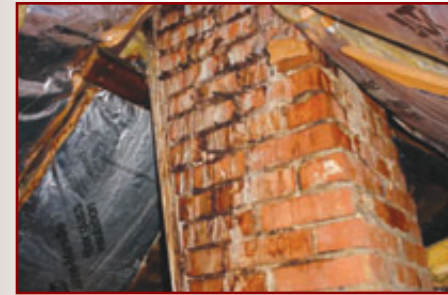
Deteriorating Chimney
